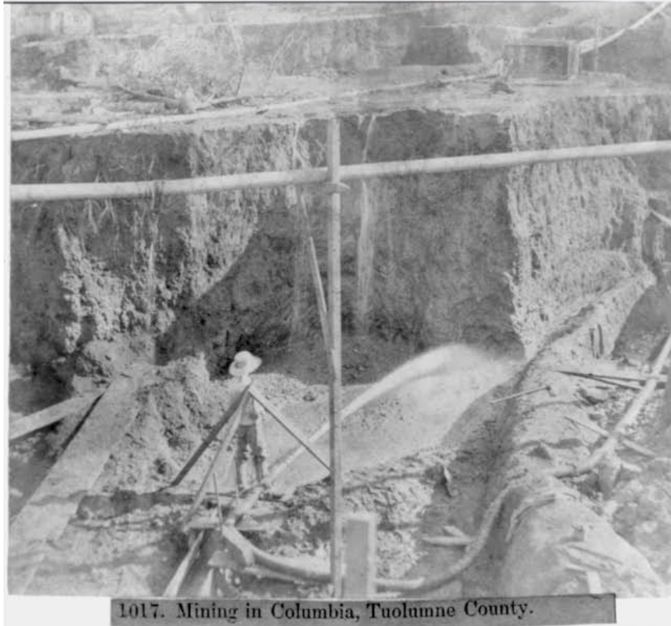
Figure 10.6 Hydraulic mining in the town of Columbia. Thousands of tons of sediment were washed from such operations into local streams and rivers, wreaking environmental havoc and property damage downstream.
