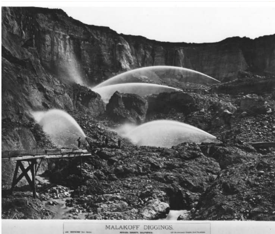
Figure 10.7 Malakoff Diggings in Nevada County near the town of North Bloomfield. Multiple monitors remove vast amounts of sediment from the hillsides and mobilize it into the south fork of the Yuba River causing major problems downstream. This operation was the impetus for the Sawyer decision that banned hydraulic mining in 1882. Runoff from the diggings continues to impact the Yuba River. From http://www.calisphere.universityofcalifornia.edu/
