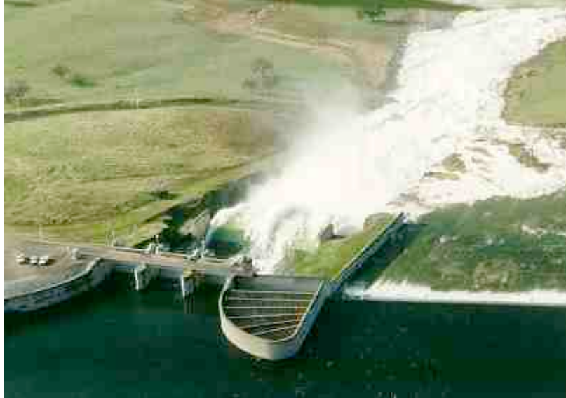
Figure 12.4 New Don Pedro Spillway during January, 1997 flood when flow reached 60,000 cfs (from Jay Lund's dam website)
