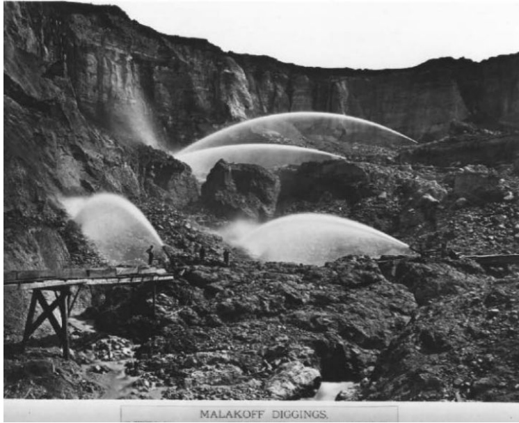
Figure 1. Malakoff diggings in Nevada County. Example of hydraulic mining during the Gold Rush. Runoff from the mining continues to impact the Yuba River. 1882
